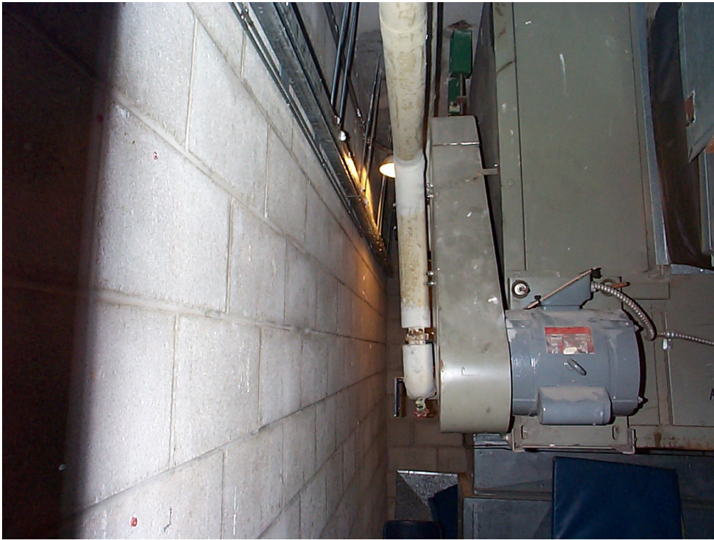
Picture #3 Furnace Room (Space #33a) ACM Elbows
